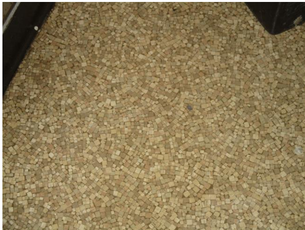
Tan Asbestos-Containing Sheet Vinyl and Associated Tan Asbestos-Containing Mastic
