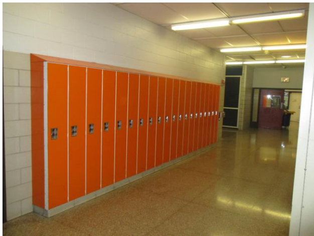
Orange Lead-Based Painted Lockers
