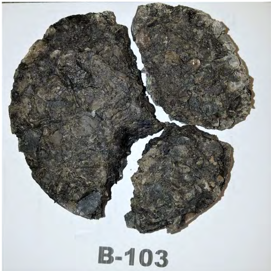
Photograph 4: Boring B-103 Asphalt Core (Bottom view of binder course)
